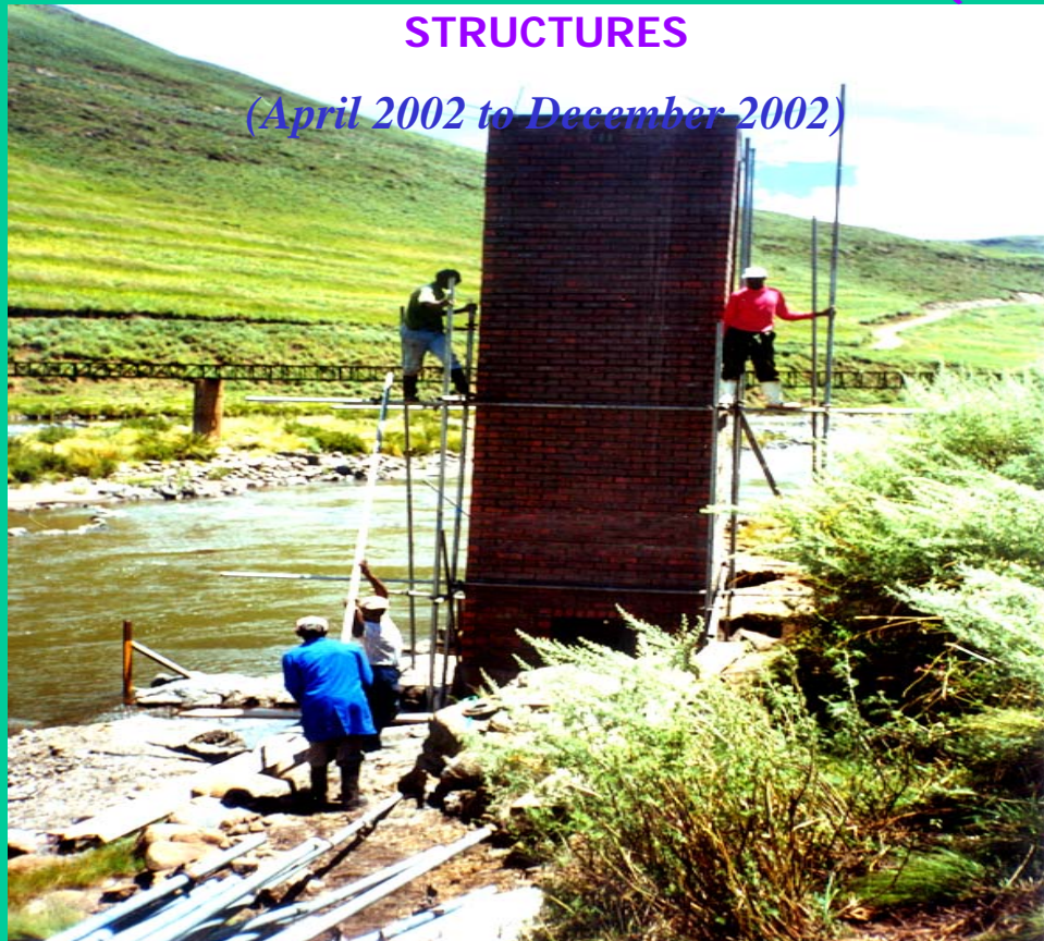
TOWER ON MALIBAMATŠO RIVER @ KAO
