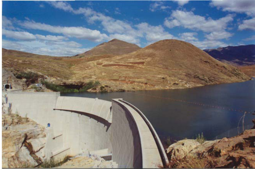
'Muela tail pond on Nqoe river. Receptacle of water from 'Muela Hydropower Plant, back into the tunnel for onward transfer to the Republic of South Africa.
