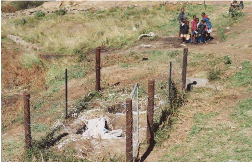
Solid wastes are fenced in and covered with soil. Just outside is the soakway concrete pit for sullen water disposal. (every household upstream of the reservoir provided with the facilities)
