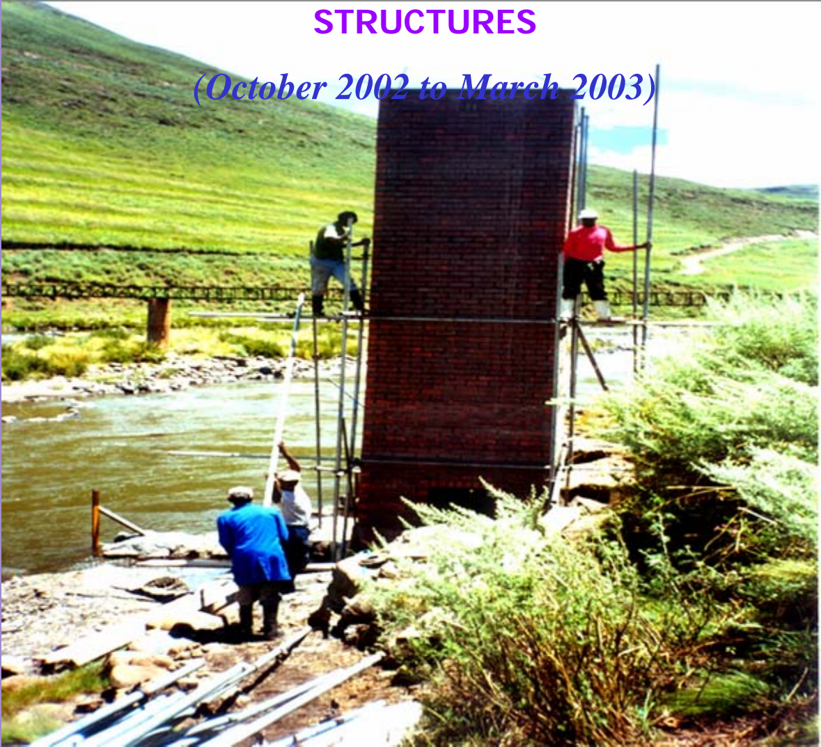
TOWER ON MALIBAMATŠO RIVER @ KAO
