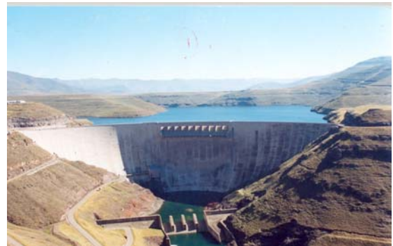
Katse Dam: Lesotho Highlands Water Project
