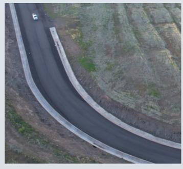
The Northern Access Road (NAR) has been repaired, including existing bridges and resealed using asphalt and minor safety upgrades. The section that has been rehabilitated stretches for 98 kilometres from the Pitseng village up to Katse village. It provides access to the Katse Dam basin and will tie into the PWAR at Ha Seshote to provide a further link to the Polihali basin.
