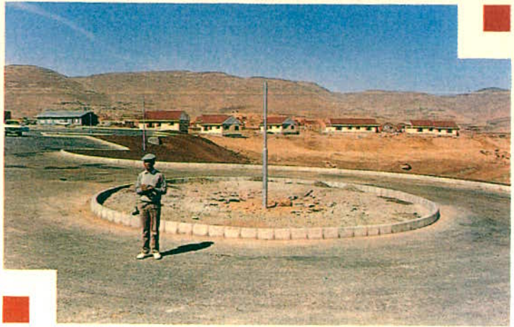
Part of the Katse Village showing progress achieved.
