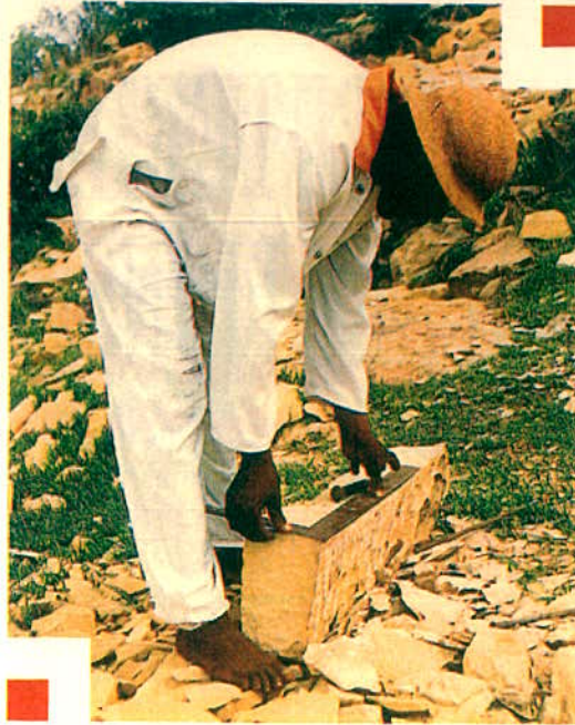
A trainee in stone masonry at work.
