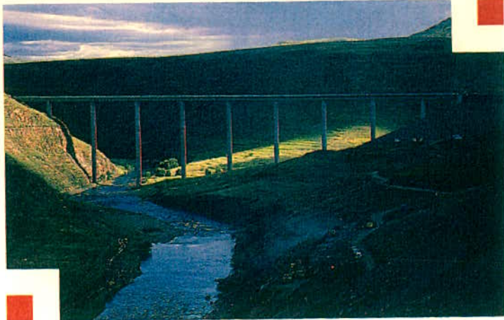
Katse Dam Site
