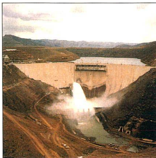
The Katse Dam releasing compensation water for downstream areas.
