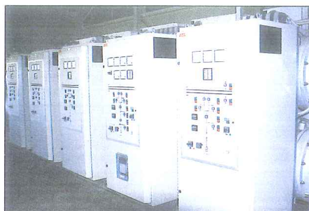
Control cubicles for power generators at 'Muela
