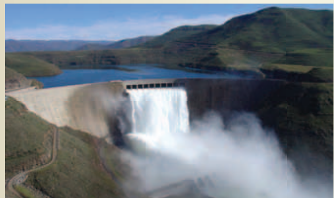
Katse Dam Spilling in November 2006
