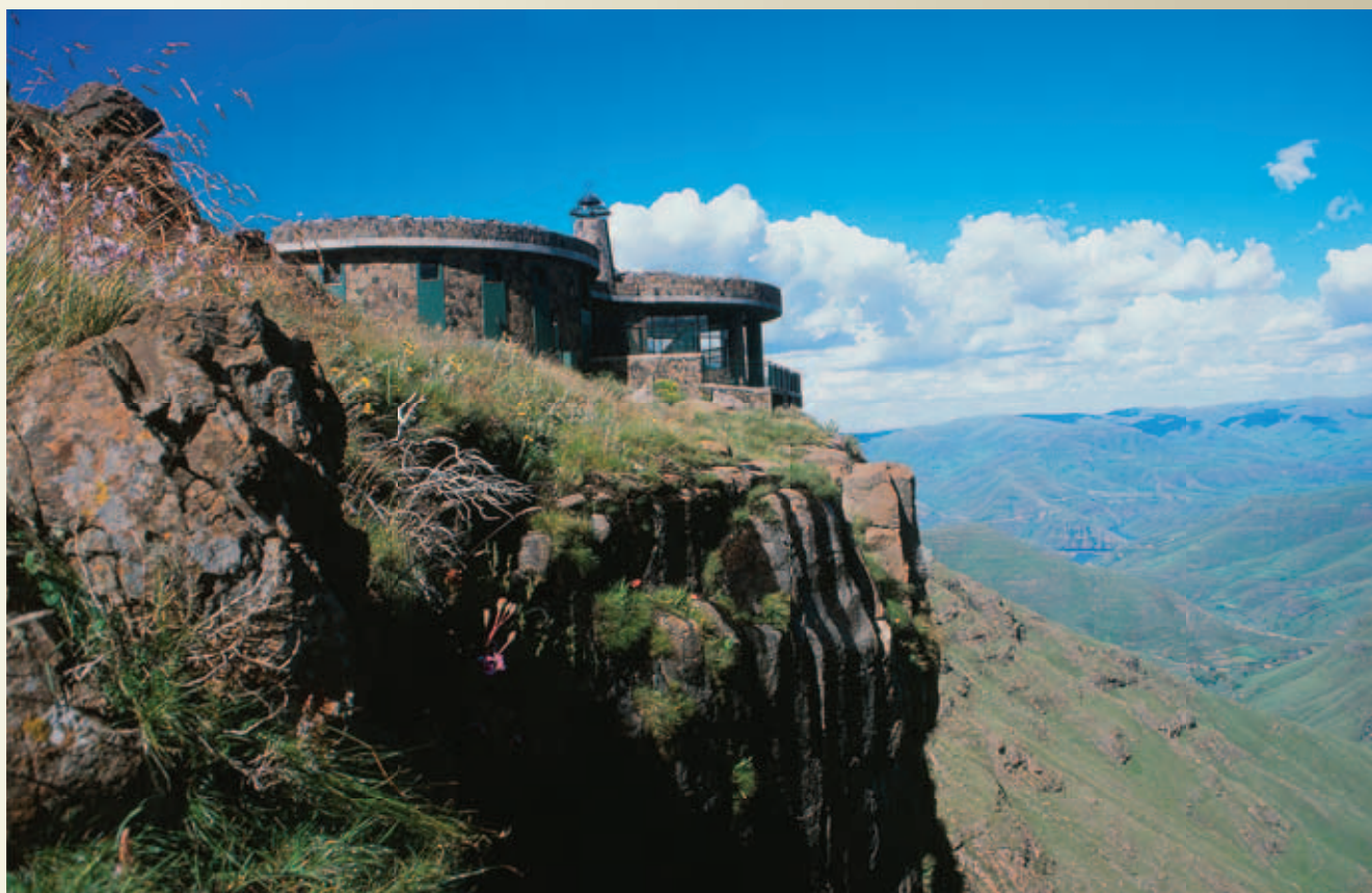
Erected at the cliff edge in a breathtaking environmentally friendly manner, the Bokong Visitor's Centre is one of Lesotho's best tourist attractions.
