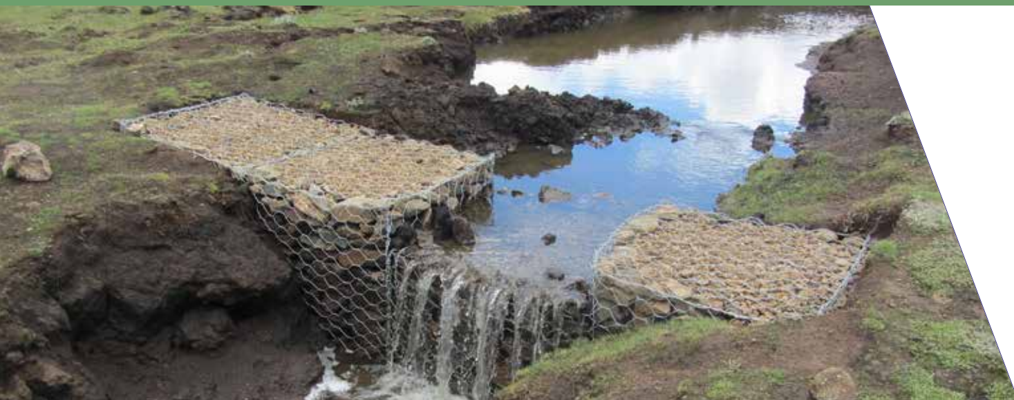
Gabion structure constructed on the Mohloathomo wetland damming back the water to allow soil settlement.
