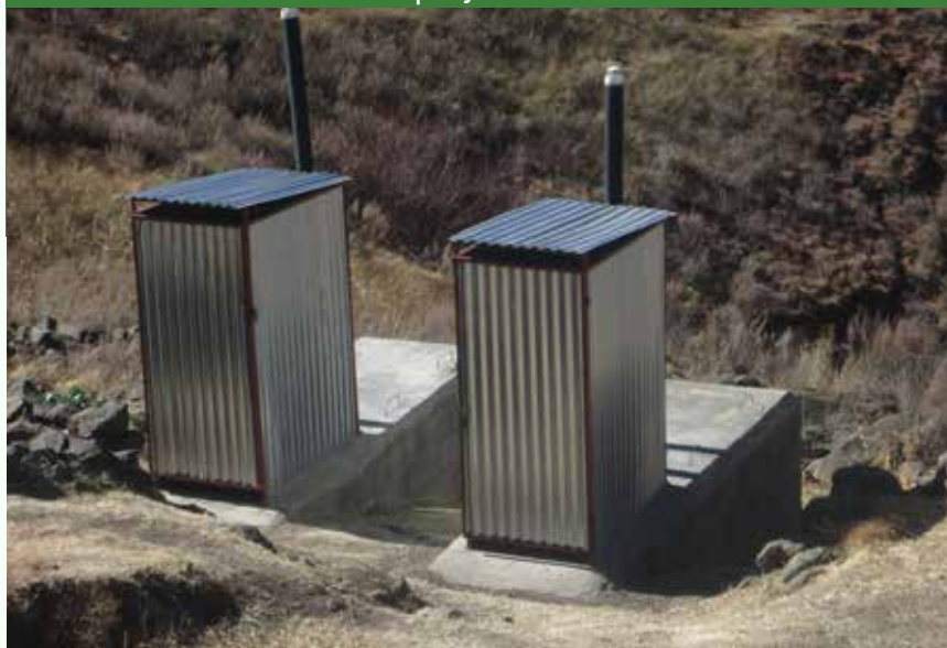
Sanitation project at Hlabathe
