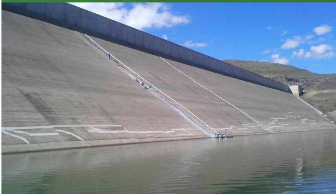
On-going repair works on the Mohale Dam face slab
