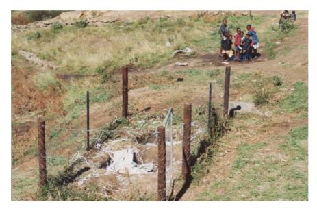
Solid wastes are fenced in and covered with soil. Just outside is the soakway concrete pit for sullen water disposal. (every household upstream of the reservoir provided with the facilities)
