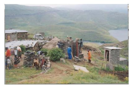
Construction of VIPs will ensure privacy for the user, address hygiene issues .They are provided with water bottles on the exterior sides for hand-washing after use of toilet. Construction of VIPs also addresses pollution coming into the reservoir from the catchment.
