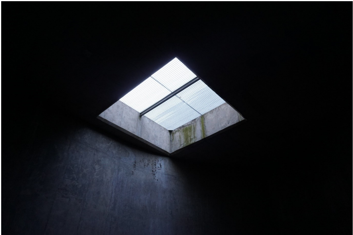
Figure 13. Access into the intake structure through the roof slab
