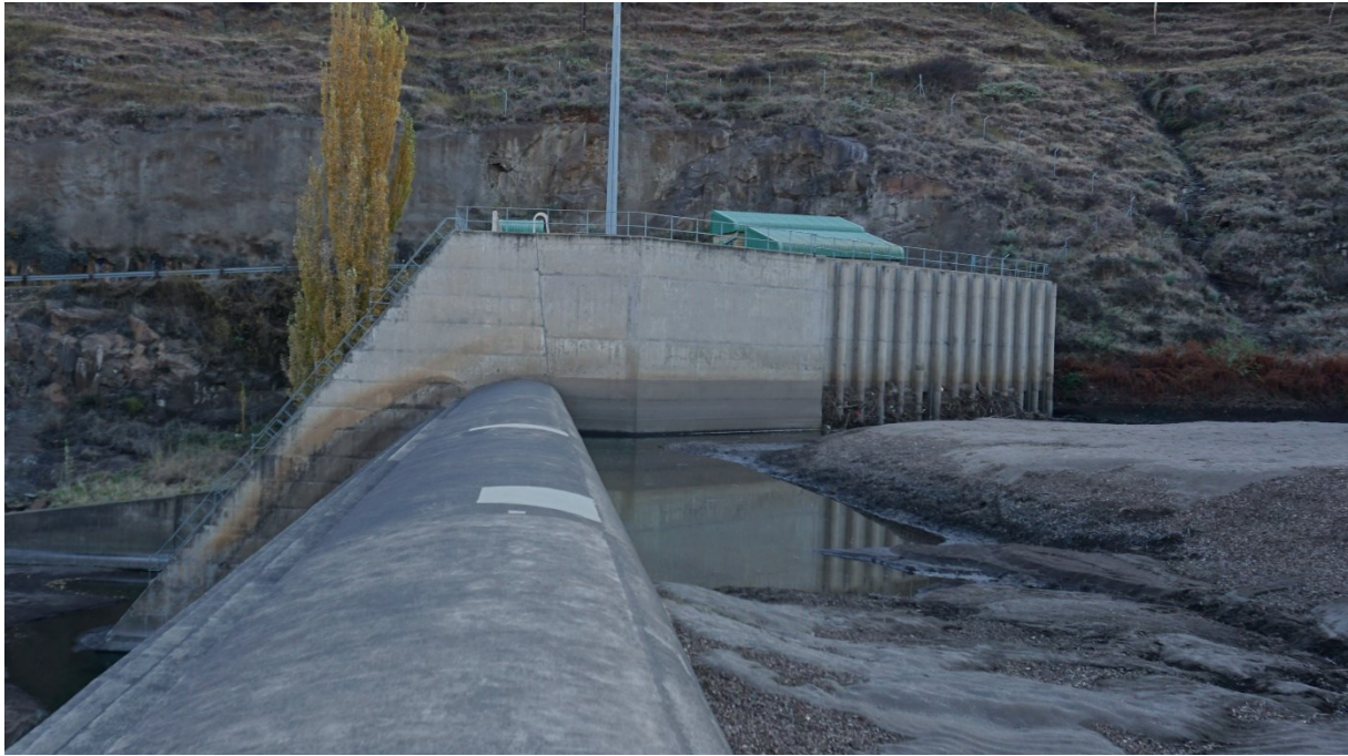
Figure 2. Matsoku Weir and Tunnel Intake Structure (7 June 2022)
