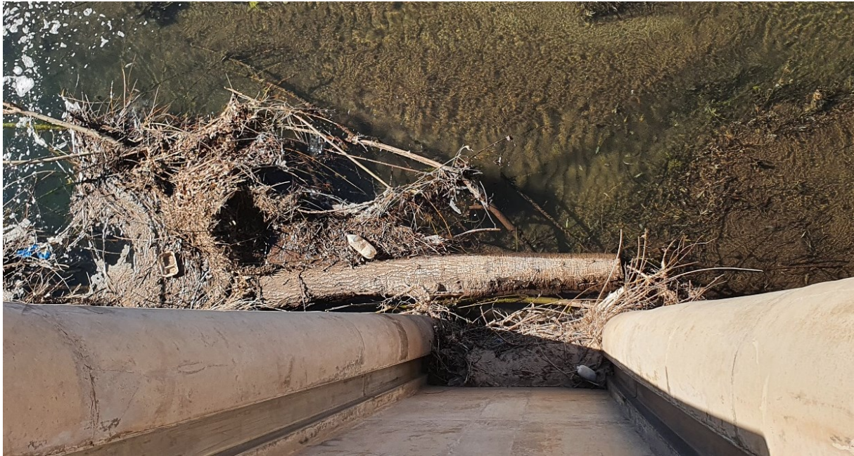
Figure 4. Top view of screen blinding (7 June 2022)
