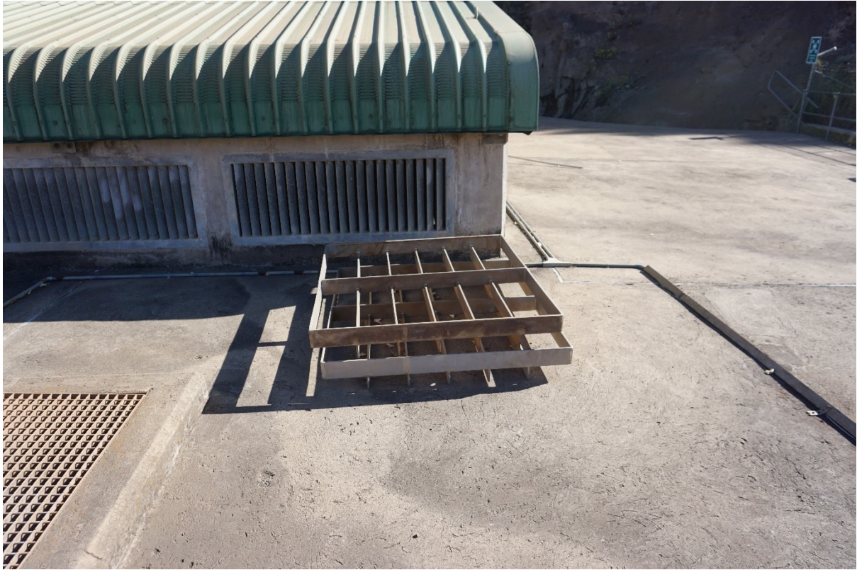
Figure 12. Two bar screen panels removed from the intake structure
